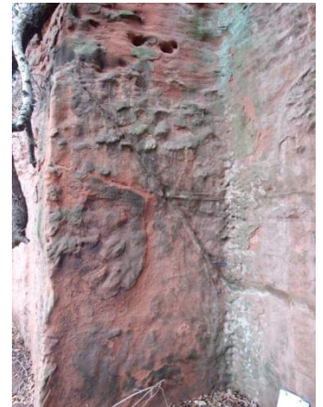
A rectangular cut into the quarry face, demonstrating a 'discontinuity' surface dipping away from the face.
