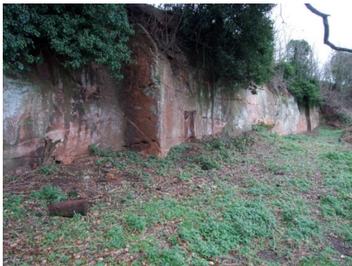
The main face of Nubbins Quarry showing how the site was worked with a vertical face, cut very smooth.
